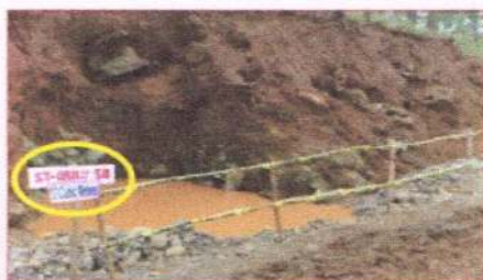
Silt trap (left) and silt pond (right) in Pimmagong.
