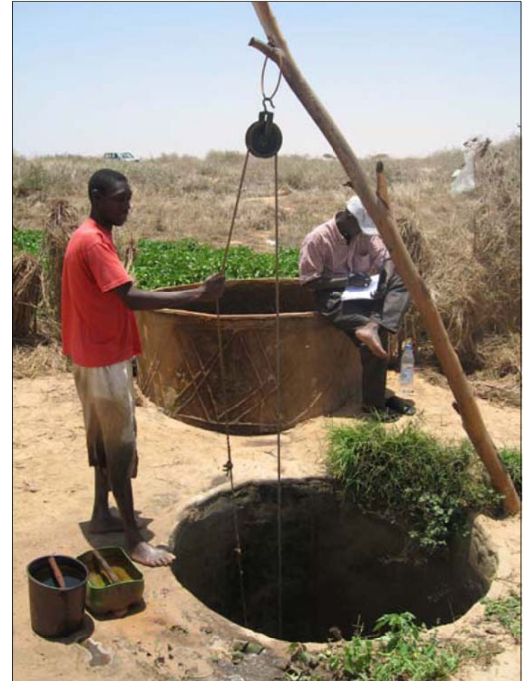
PLATE 4.2 Typical private well with holding and distribution vessel in background Source: Earth Systems Pty Ltd, Melbourne (2010)
