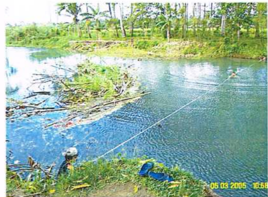
Photo 5-2. The wide river channel of Magpayang River where Harrison Bridge that connected the National Highway to Brgy. Siana used to stand.
