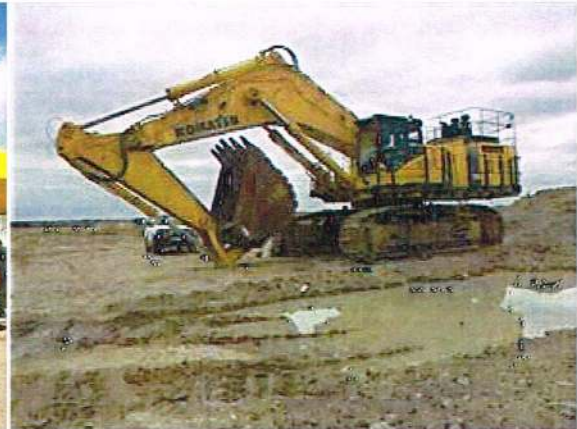
Photo 3-6. The Komatsu Excavator PC1250-7 with 5 m 3 bucket capacity.
