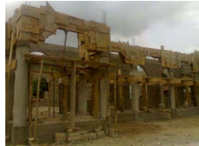
Construction of new mosque in Bumbuna currently underway
