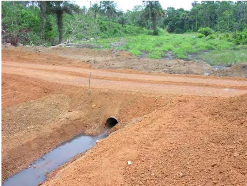
Figure 9-1 Example of a flume pipe access
