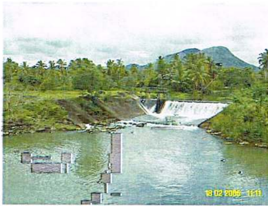
Photo 3-31. The irrigation dam at Magpayang River for Brgy. Magpayang immediately upslope of the dilapidated bridge (BMP, 2009).
