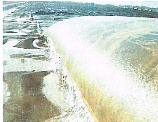
Photo 5-5. Clean and clear water drips out of a geotextile tube (J.R. Wynn).
