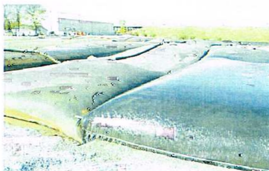
Photo 3-39. A typical layout of geotextile tubes in a construction site.
