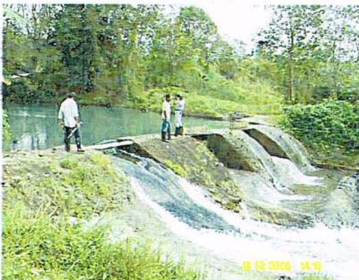
Photo 3-33. This irrigation dam at Dayano Creek services the rice fields of Brgy. Siana (BMP, 2009).
