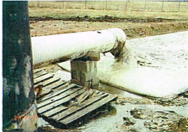
Photo 5-3. Filling of tubes by gravity method (J.R. Wynn).
