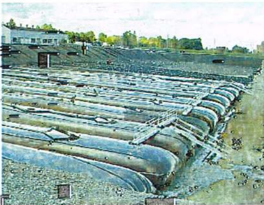
Photo 5-4. A geotextile tube farm (J.R. Wynn).
