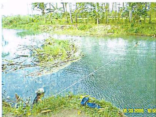
Photo 3-29. The wide river channel of Magpayang River where Harrison Bridge that connected the National Highway to Brgy. Siana used to stand.
