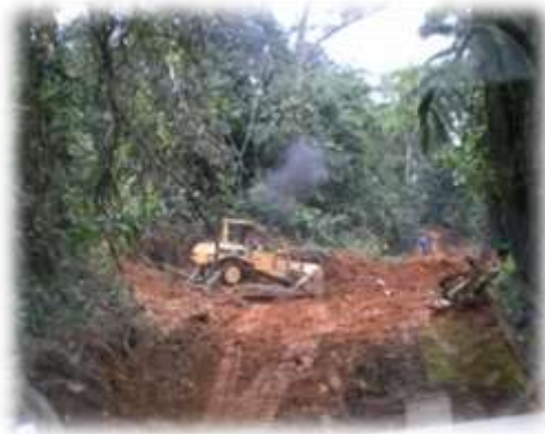
Above: Earth moving activities (GroundTruth 2011)
