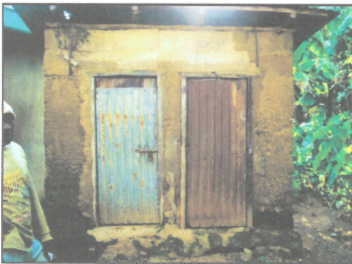
Photo 7: Pit latrine constructed with bricks
