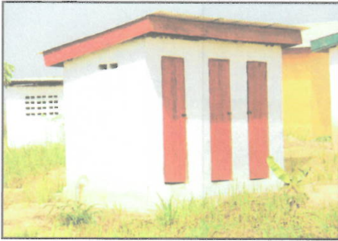
Photo 30: Example of newly constructed VIP toilet in resettlement village
