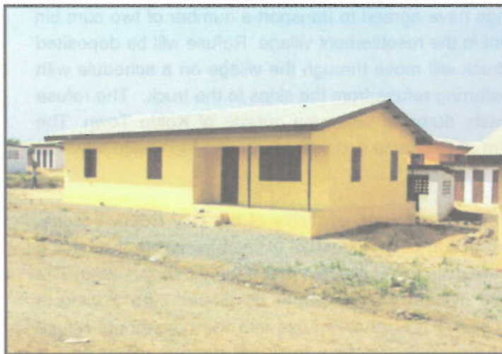
Photo 29: Example of a replacement house in the Koidu resettlement village
