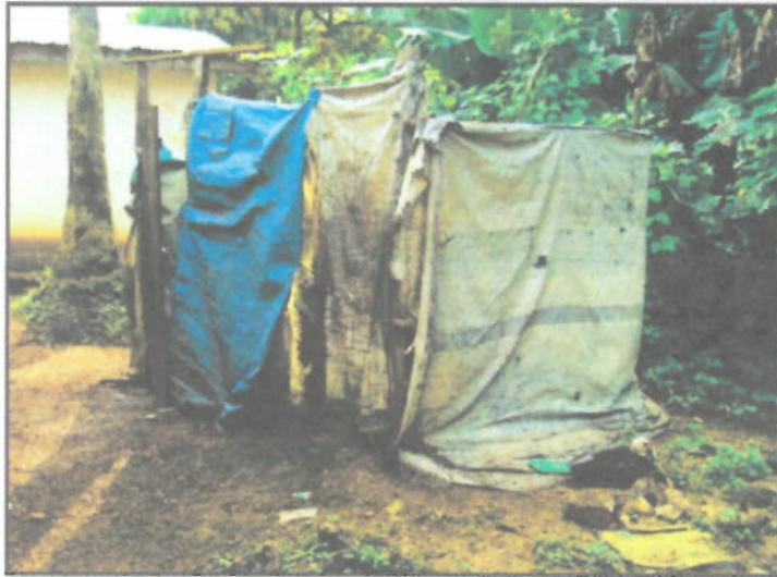
Photo 6: Pit latrine constructed with plastic sheets
