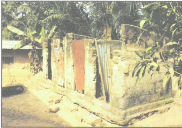
Photo 11: Typical pit latrine structure in villages
