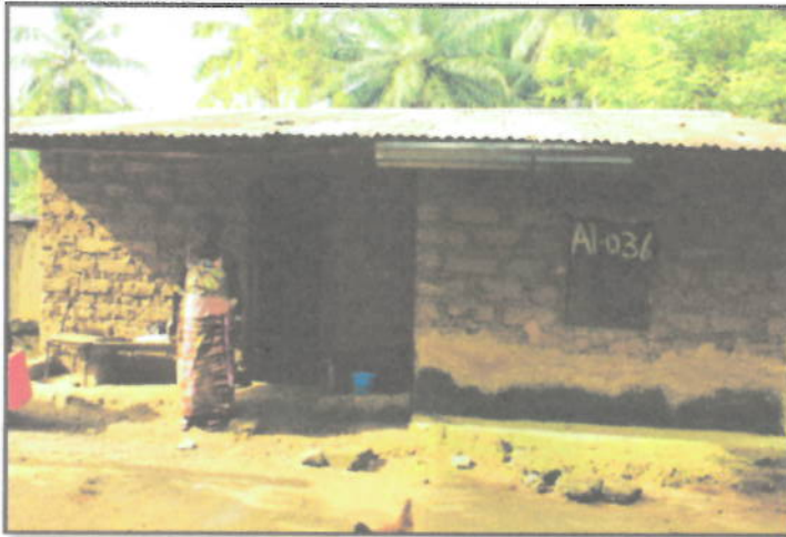
Photo 4: House constructed with mud bricks
