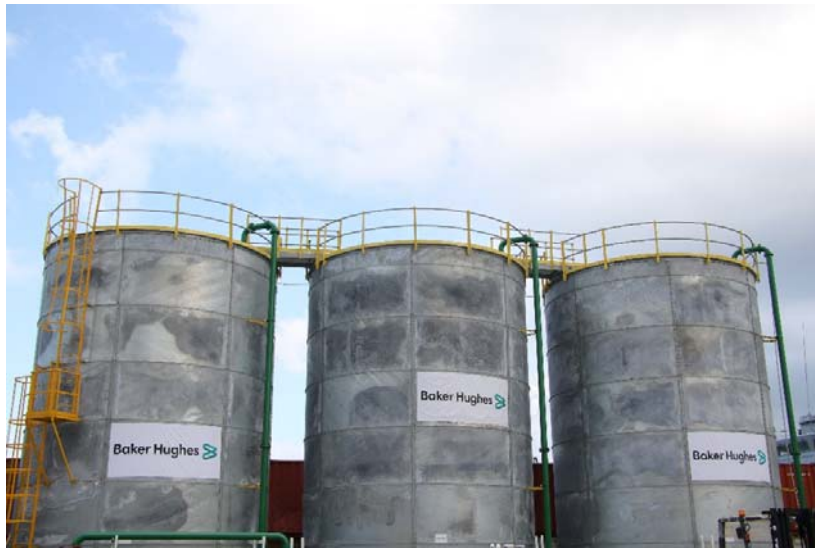
Figure 4.9: Photographic example of a drilling fluids mixing plant
