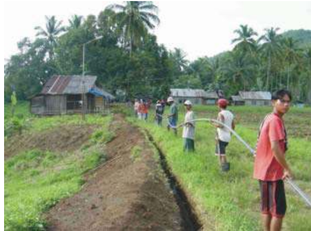
Photo 3-6. Pipe laying by the barangay residents.
