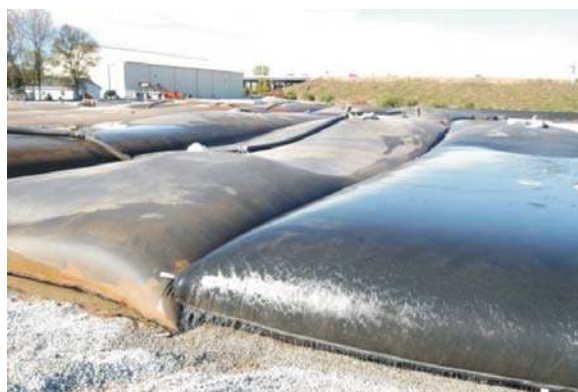
Photo 3-25. A typical layout of geotextile tubes in a construction site.
