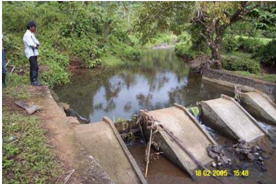
Photo 4-19. The small irrigation dam across Cawilan Creek.
