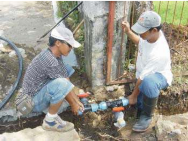
Photo 3-7. GRC staff fixes the pipe network.
